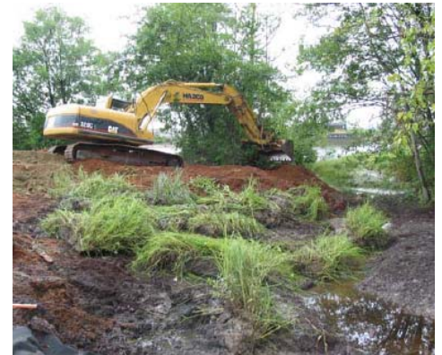
Ditch Realignment Construction Phase
